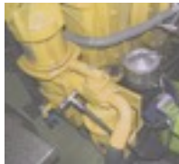
Triple R installed on existing line
